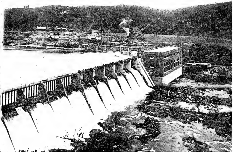
FIG. 35.—Typical Masonry Dam of the Gravity Type. Appalachian Power Company.
